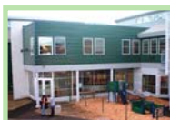
Cross Roads House Portsmouth
