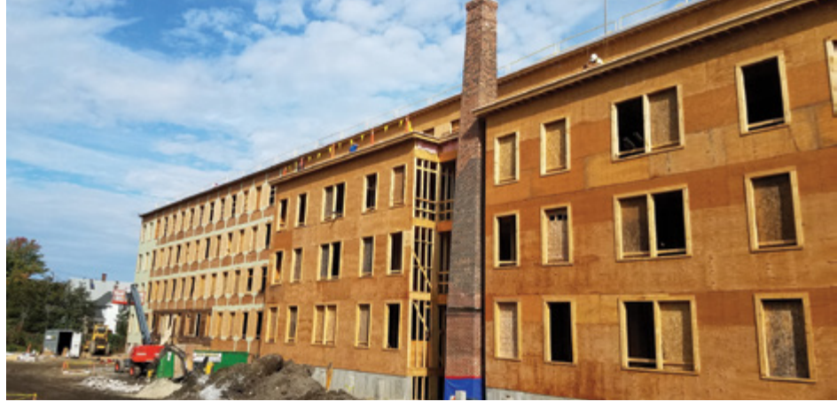
Ivory Keys Apartments under construction
