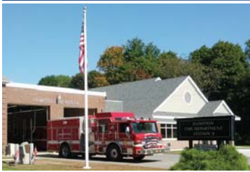
Hampton Fire Station #2 Hampton, NH
