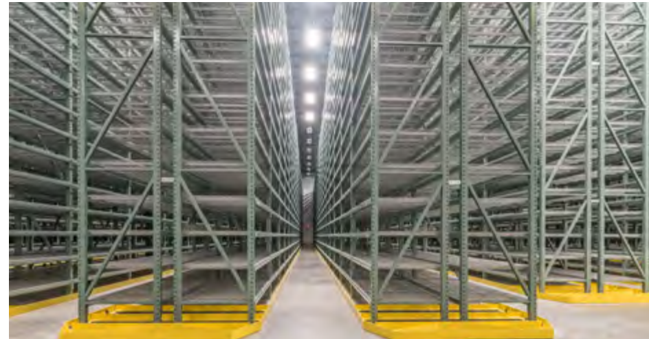
Interior of the specialized racking system that will house all of the volumes
