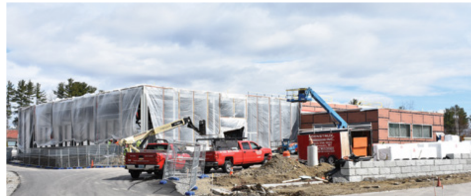
Land Rover facility under construction
