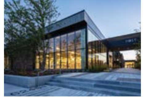
Redesigned office building / photos courtesy of Anchor Line Partners
