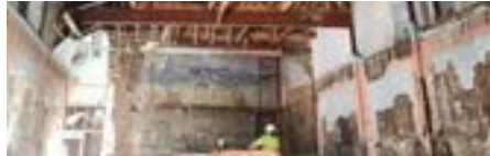
Concord Theatre renovation in progress
