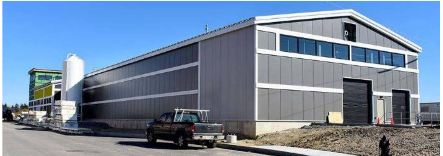
603 Brewery and Restaurant under construction
