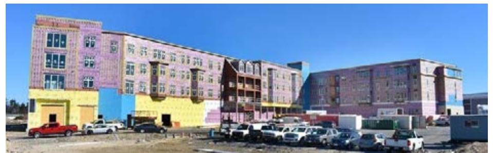
Phase 1 at Woodmont Commons under construction
