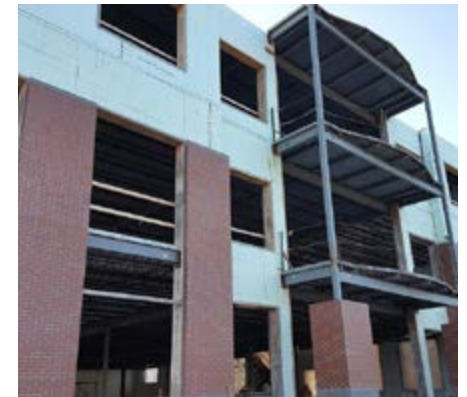
Construction showing exterior ICF walls and steel framing
