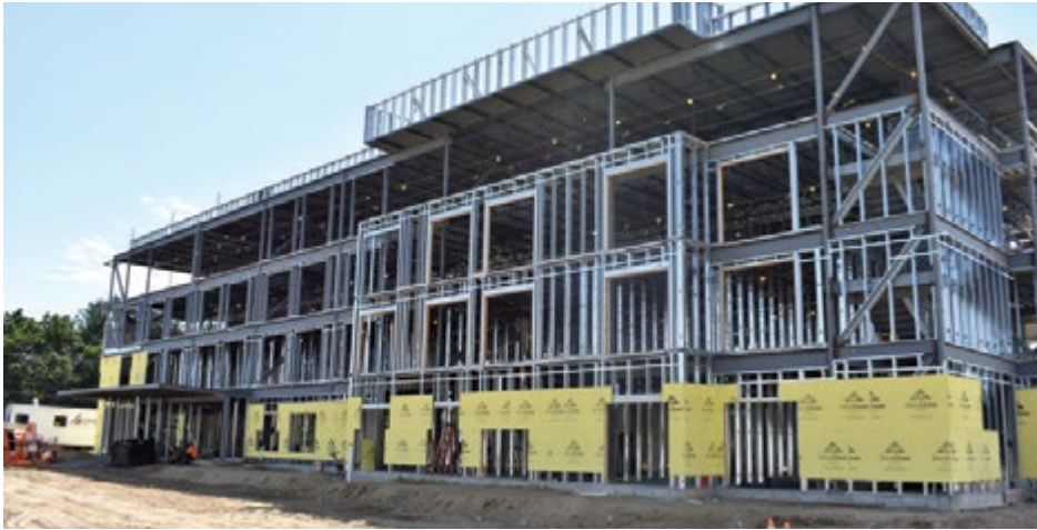
Tru by Hilton under construction
