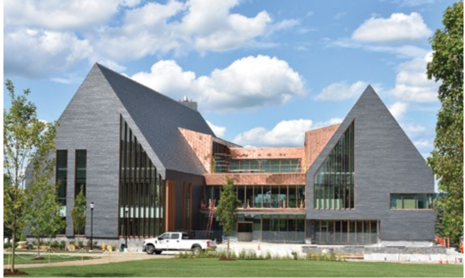
CETA under construction
